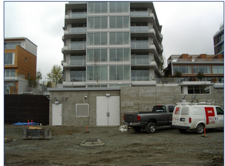
Dockside Green treatment plant
